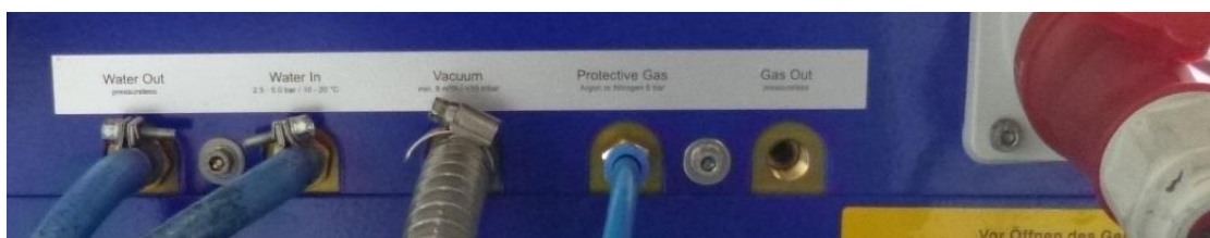
Figure 35: Check of the backside connections
